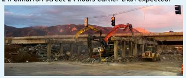
The I-25 bridge crossing over Cimarron Street/US 24 is the largest bridge demolished on the I-25/Cimarron Interchange Design-Build project. The ability to temporarily close Cimarron Street/US 24 under the interstate for quick demolition saved what would otherwise have required several weeks (2-3) of overnight closures had the old bridge been removed in pieces. Not only that, but implementing a full weekend closure resulted in a much safer operation and guaranteed quality work.
